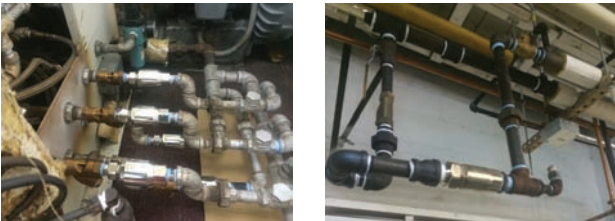
Apollo Trap Installation
